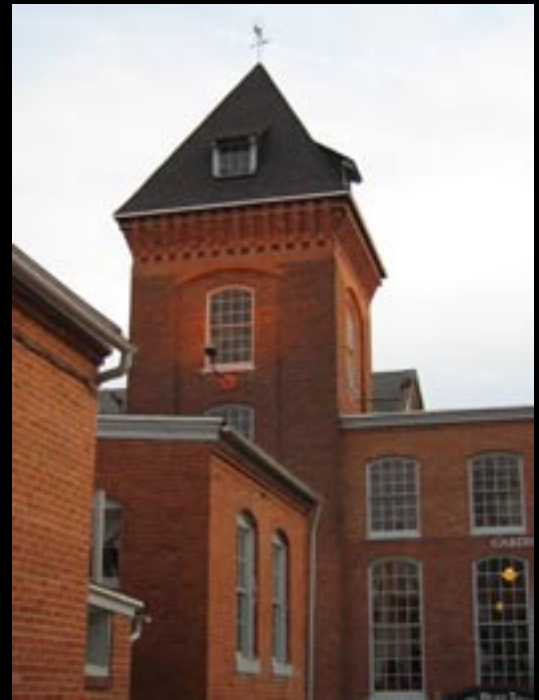
Savage Mill Tower - The tower is only one of several spots in this 19th century site reputed to be haunted. Among other sightings, the ghost of a woman who fell down the stairs to her death has been seen here for decades.
